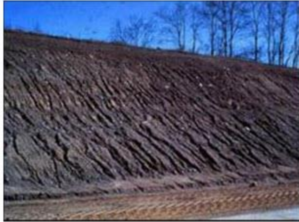
Fig. 3.3. Rill erosion. (Source: http://www.kalkaskacounty.net )
