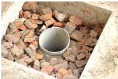
Filter materials in a soakaway
