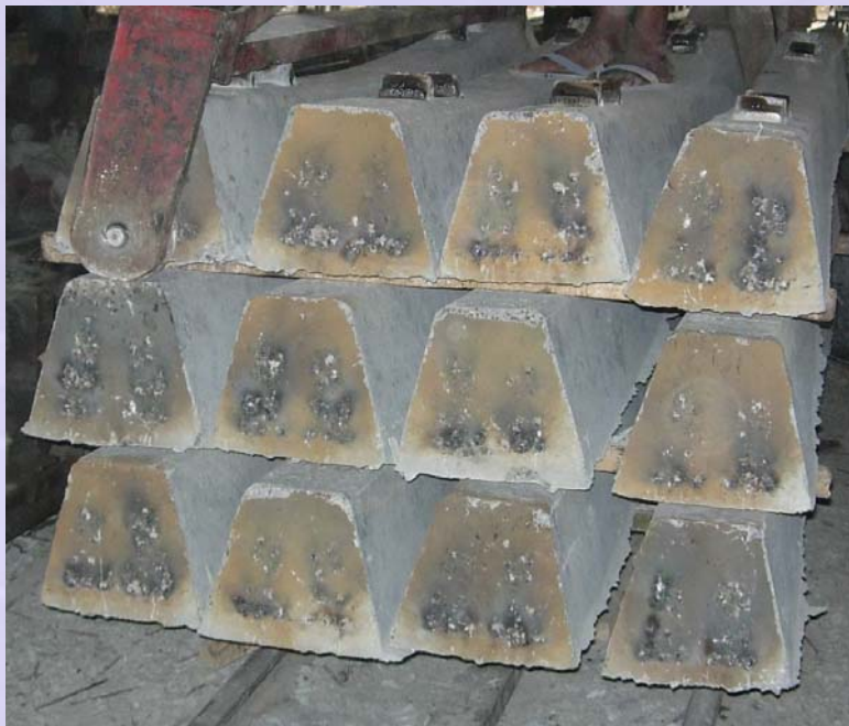
Figure 7-1.1 End of pre-tensioned railway sleepers
